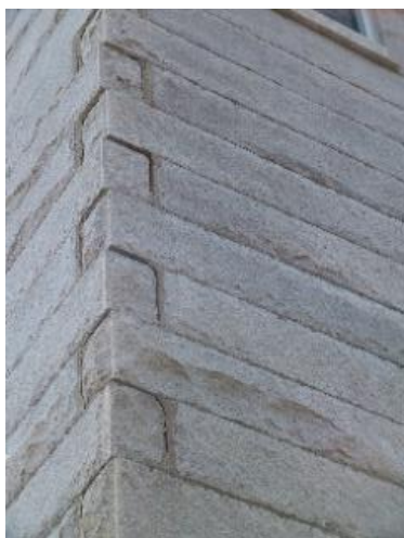
Expansion of the Granite Quoins from Frozen Exposures
