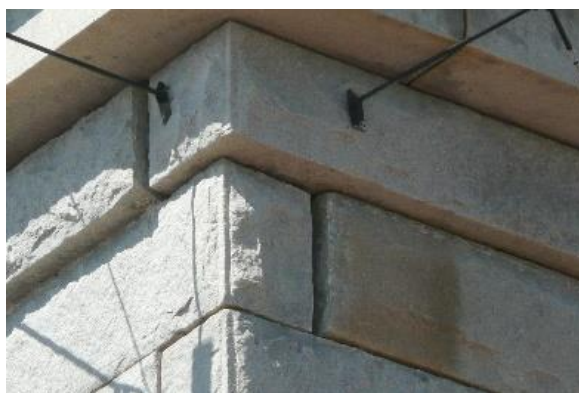
Expansion of the Granite Quoins from Frozen Exposures
