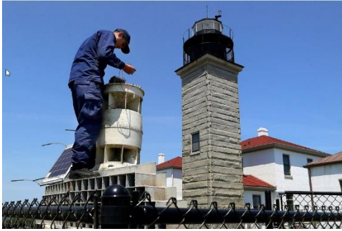
US Coast Guard Technician, Rocky Recio, from Bristol ANT, repairing the fog signal.
