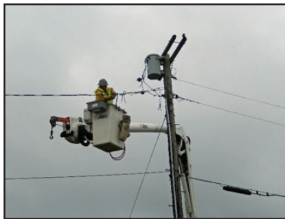
National Grid cutting overhead cable
