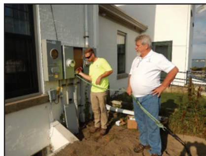
Feeding cable into conduit
