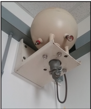
A "new" display: Halon 1301 fire suppression system sphere in the Tower Control Room..
